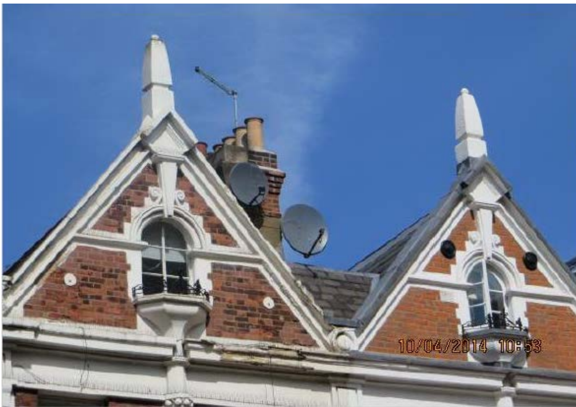
View of infill extension at roof level to front elevation.
